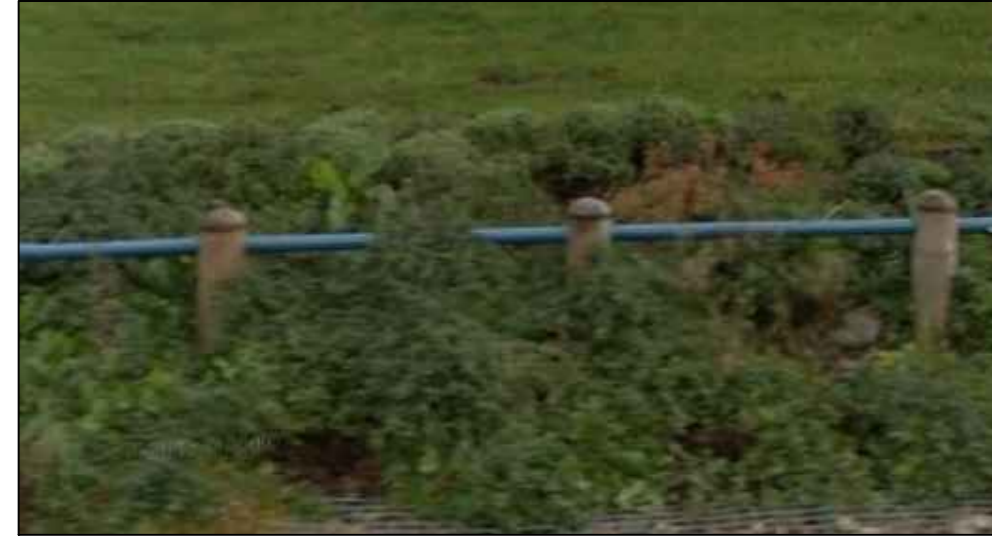
LOW TIMBER BOLLARD & RAIL
